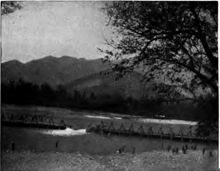
First breach in the 'barrage' at Kwanhien (to be followed by its total removal), whereby the waters of the Min are admitted into the hitherto dry North-eastern irrigation system. This 'barrage' is removed each year in April and replaced again in November.
